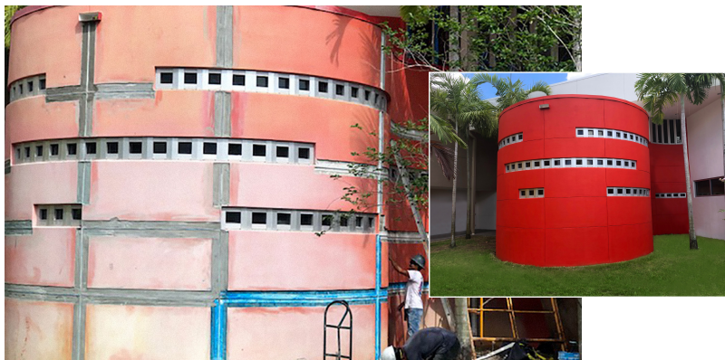
Jewish Adoption and Family Care Options, Ft. Lauderdale, FL, stucco surface prep (left) and completed (right)
