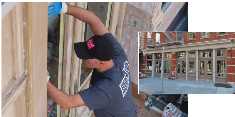
New York City, NY, Store Front (56-58 Warren Street) wood surface prep (left) and completed (right)
