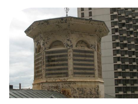
Peeling paint, corrosion, and general deterioration of the cupola was extensive.
